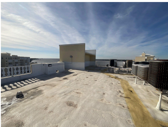
Typical flat roof
