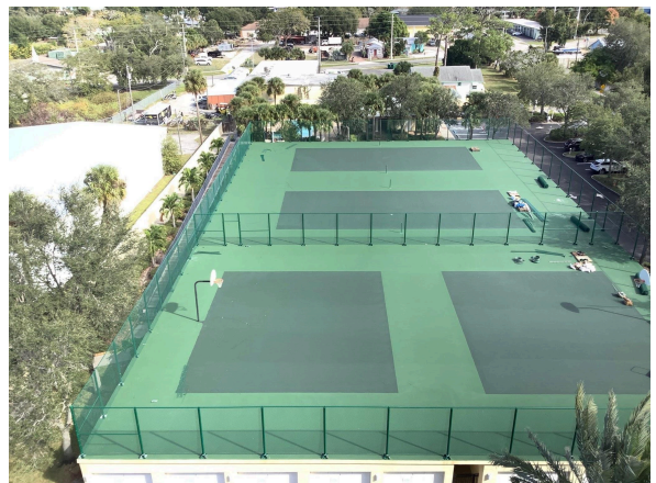
Sports courts on garage - upgrades in progress
