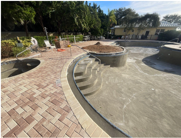
Clubhouse pool area - resurfacing in progress
