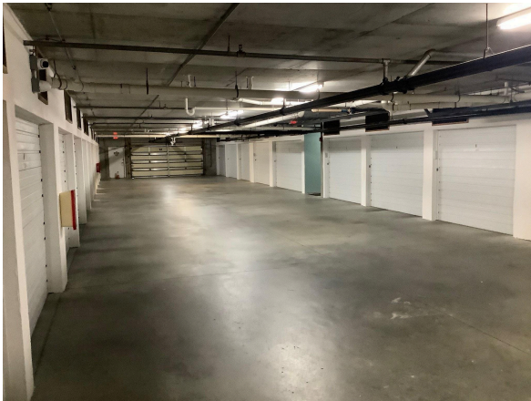
Typical parking garage
