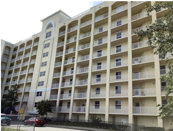
Typical building exterior
