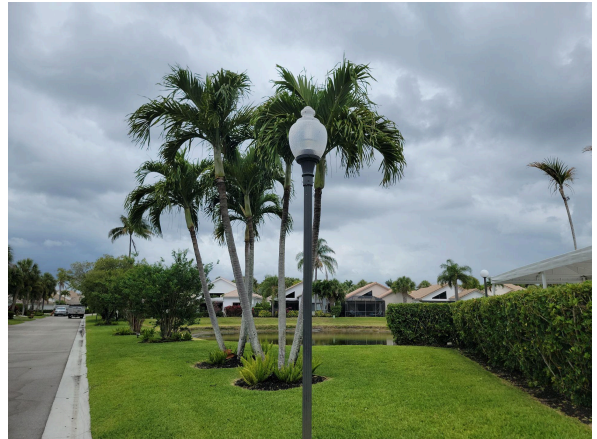
Typical street light
