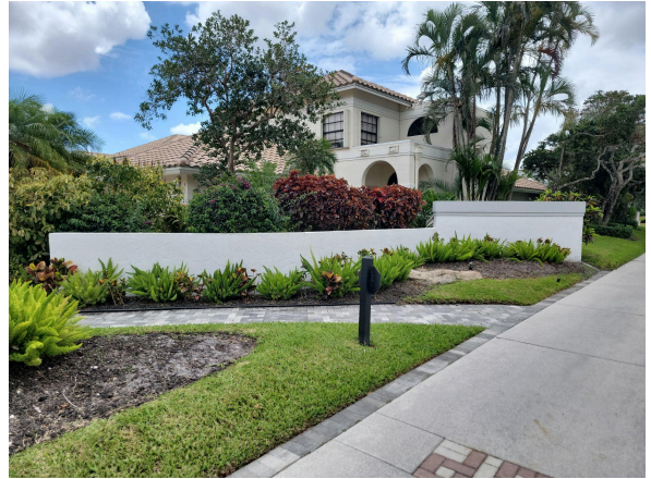
Stucco wall at entrance of community
