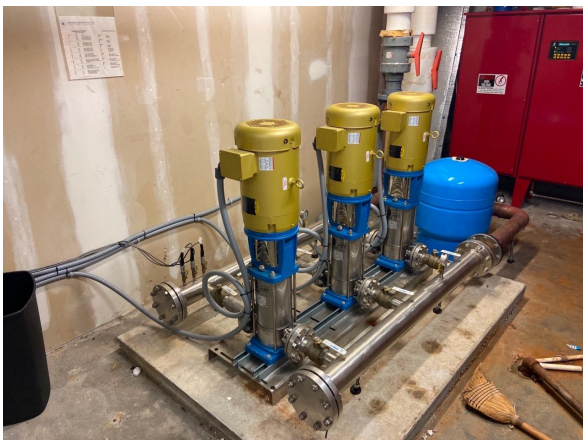
St. John fire sprinkler jockey pumps
