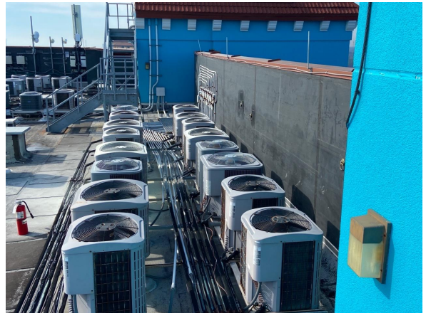
Common area HVAC condensers
