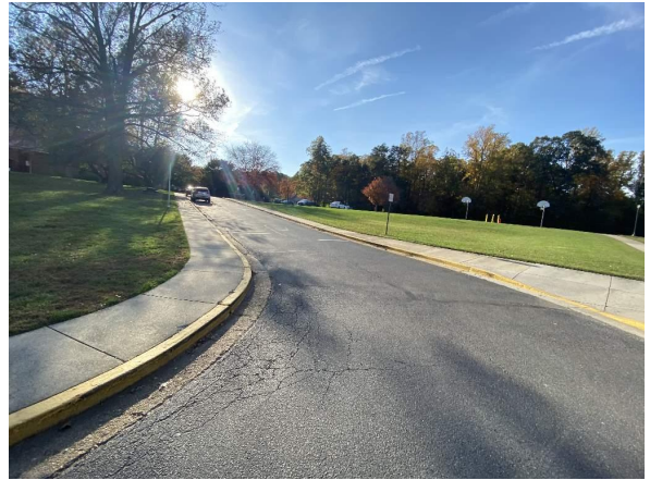
Typical condition of asphalt parking lot
